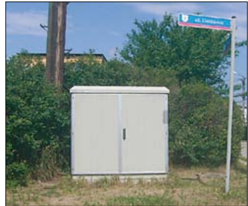
Cabinet before extension
