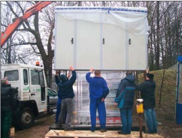
Cabinet during extension
