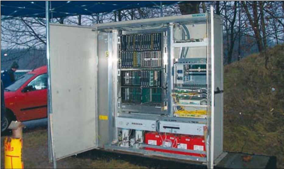
Cabinet before extension
